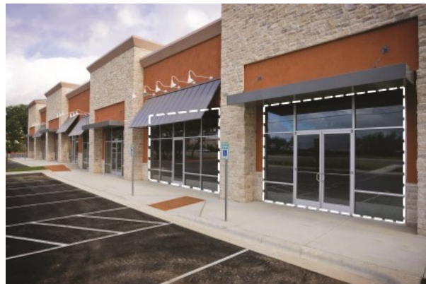
Figure 13.09-C: The window area is illustrated within the dashed line area for the two storefronts in the above image.
