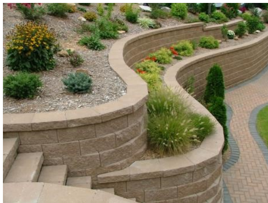
Figure 9-C: Retaining walls shall be benched, or terraced, so that no individual wall exceeds a height of six feet.
